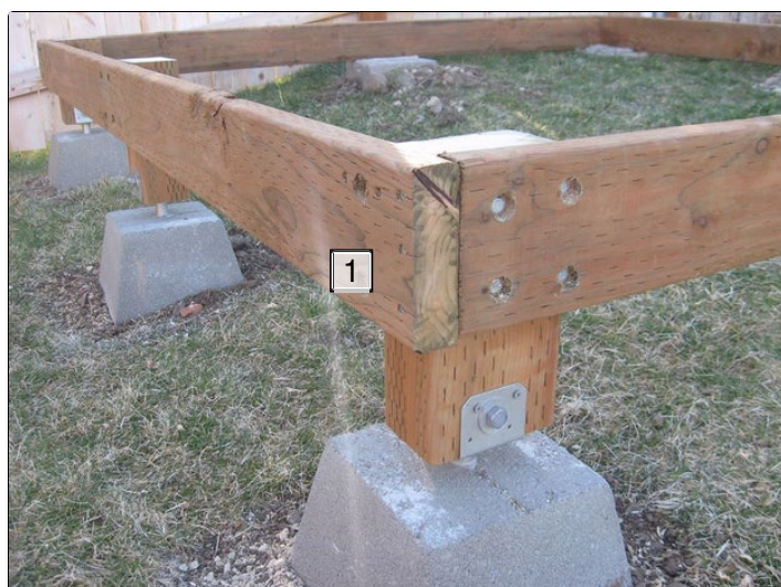
1. Holes were bored about 1/2" deep with a 1" spade bit prior to pre-drilling for the shaft of the lag bolts.
