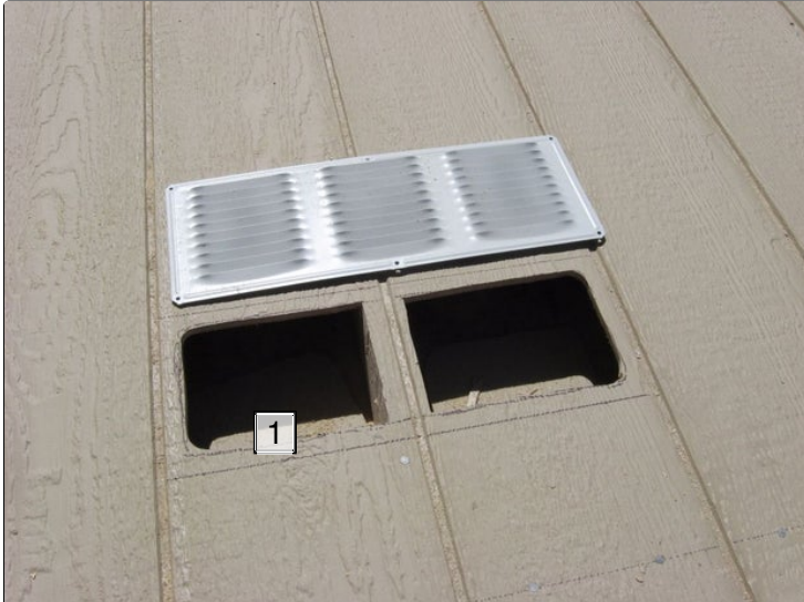
1. Openings were marked and cut with a jigsaw, and the vents screwed in place. Will actually be temporarily removed later when I paint.
