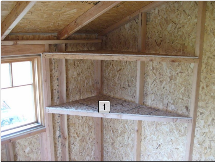
1. Pieces of OSB were screwed in place to the shelf frames.
