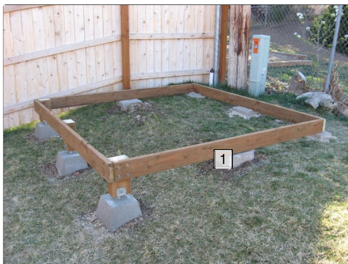
1. Note the two blocks stacked here at the midpoint. These were glued together with landscape adhesive.
