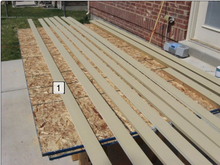
1. All trim pieces were painted prior to installing with a couple coats of 'Harvest Brown' exterior Behr paint.
