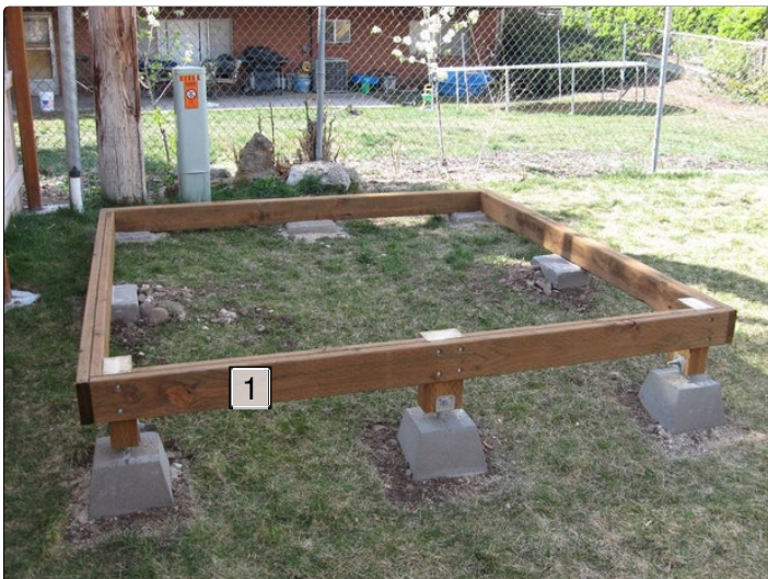
1. Finished frame is exactly 8 feet by 8 feet.
