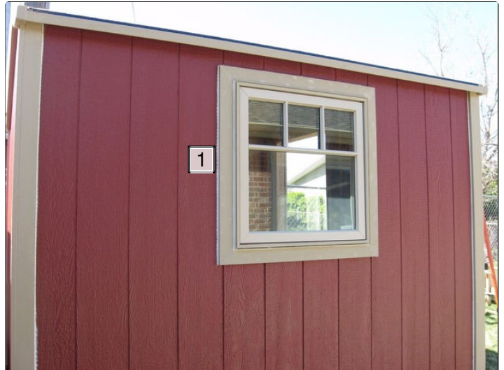
1. For exterior applications like this, caulk the sides and top, but not bottom edge (to allow moisture to escape).
