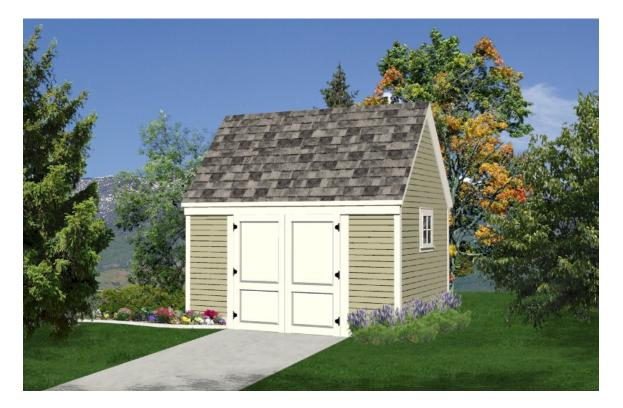
This solid, permanent 2x4 stud-frame shed, on a concrete slab foundation, has convenient lofts for additional storage.
