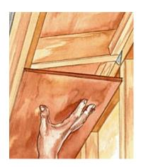
Rip the soffit panels to fit between the wall plates and fascia. Fasten the panels to the nailers, rafters, and subfascia.
