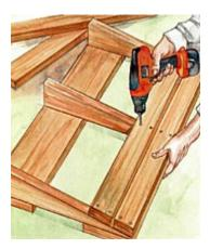
Build the ramp with pressure-treated  $2 \times 8s$  and  $2 \times 4s$ , following the plan's size or building it to a custom size.
