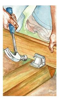
Secure the joists to the outer skids with angles. Drive hanger nails into the joists and 16d nails into the skids.
