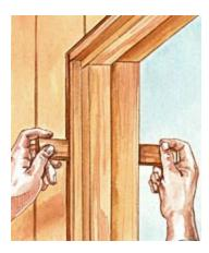
Use pairs of tapered shims to plumb and level the door frame in the rough opening.
