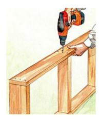
Assemble the window frames with screws. Add a  $2 \times 4$  mullion in the center of the side window frame.
