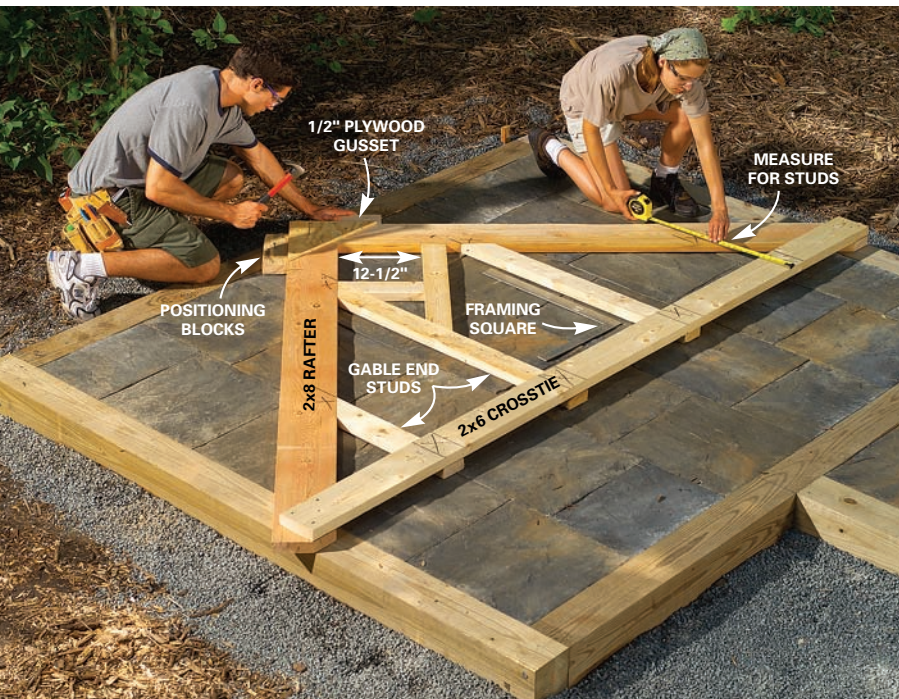
Figure C Rafter Details
